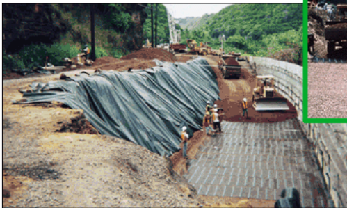
▲ Kamehameha Highway workers laying the geogrid behind the Full-Height Panels.
